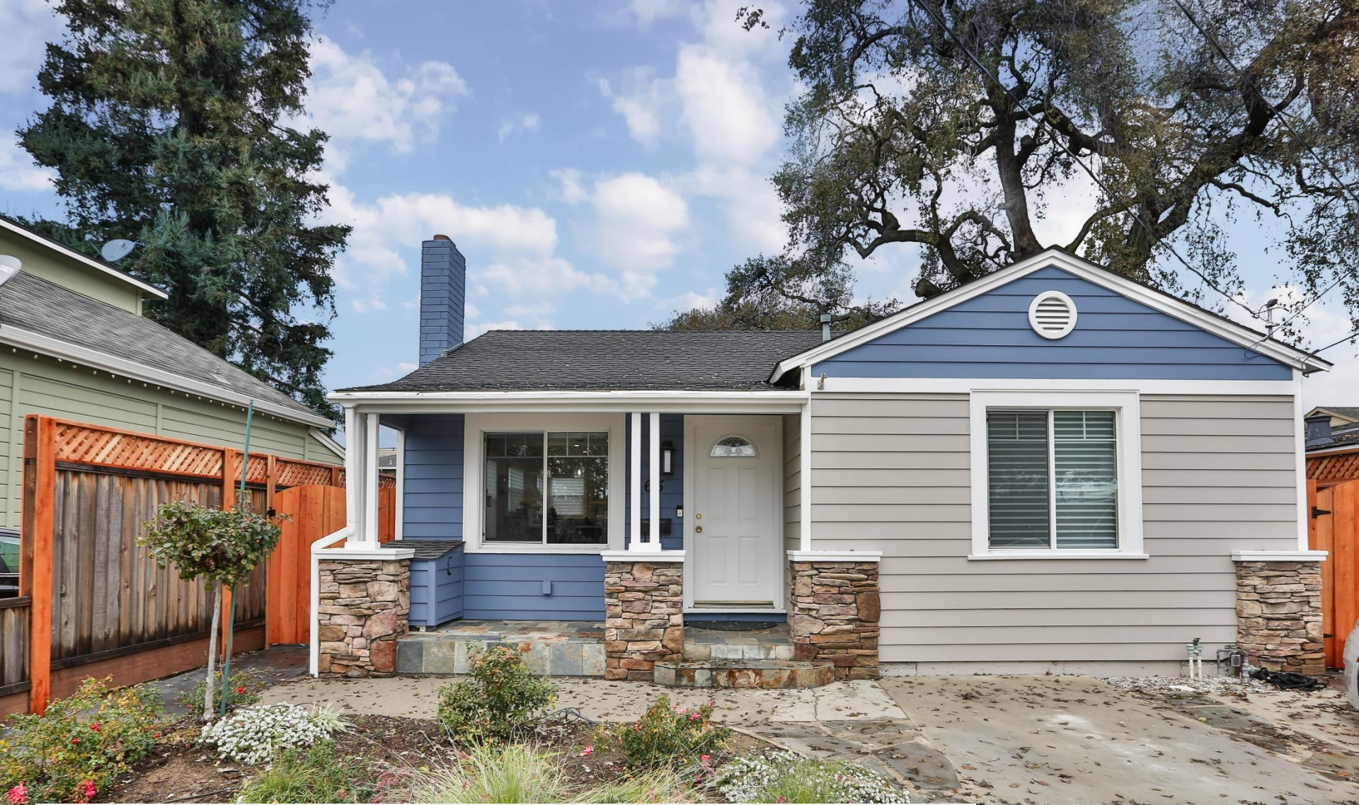
EXTERIOR AFTER: With a new, youthful paint scheme, the exterior now properly echoes the interior of the home. By extending the great room color palette outwards, the house is beautifully cohesive. The posts and window casings were replaced and repainted as well. Fence sections and gates were updated to match the existing.
