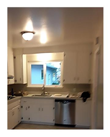
The size differential between wall cabinets surrounding window looks awkward and unbalanced. Small blind cabinets (both at base and wall cabinets) to the left of the sink had tiny openings, making access impossible even though they had interior open space.
